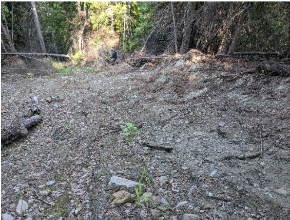
Photo 22. 5 km McGregor FSR landslide
