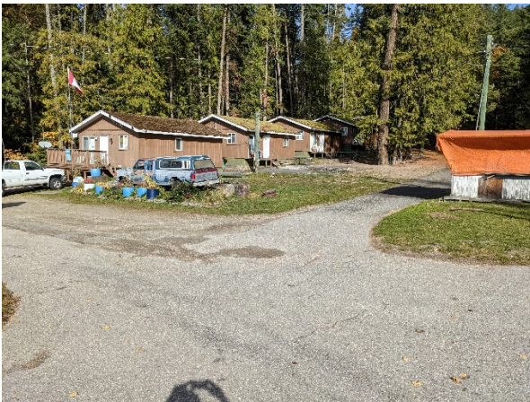
Photo 35. Cabins and office/dwelling on Lockhart Creek fan.
