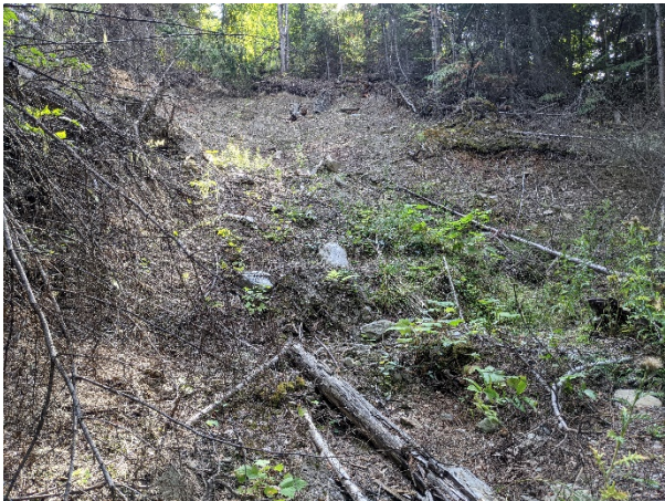
Photo 23. 5 km McGregor FSR landslide
